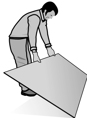
Figure 8 – Intermediate slab horizontal positioning phase
